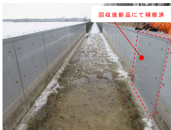
Fig.1 調査水路の外観 Appearance of surveyed channel
